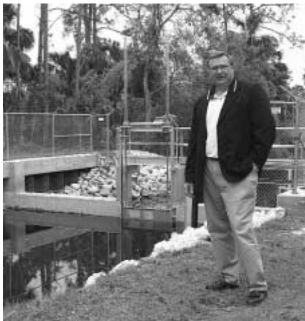
Tom Powell stands in front of the new water control structure south of Indiantown Road in Jupiter Farms
